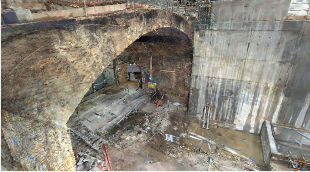
Figure 3: View of a photogrammetric model of a brick arch at London Bridge Station (Follow the link to: https://www.youtube.com/watch?v=2WXEAebFCao )
